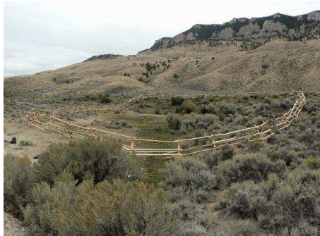
The completed buck-and-rail fence encloses nearly three acres. (Photo by John Rumm)
