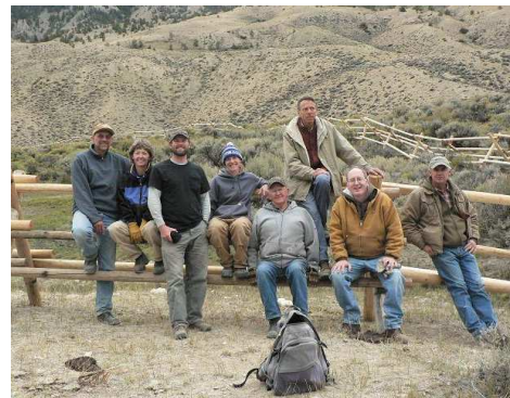
Members of the crew that built a buck-and-rail fence on Sheep Mountain in October pose for a photograph. Left to right: Mike Stokesbury, Rosemarie Hughes, Destin Harrell, John Ross, John Osgood, John Rumm, Sean Sheehan. Not shown: Dana Ross, Gordon Ross, Lyn Stallings, Alex Rumm.
